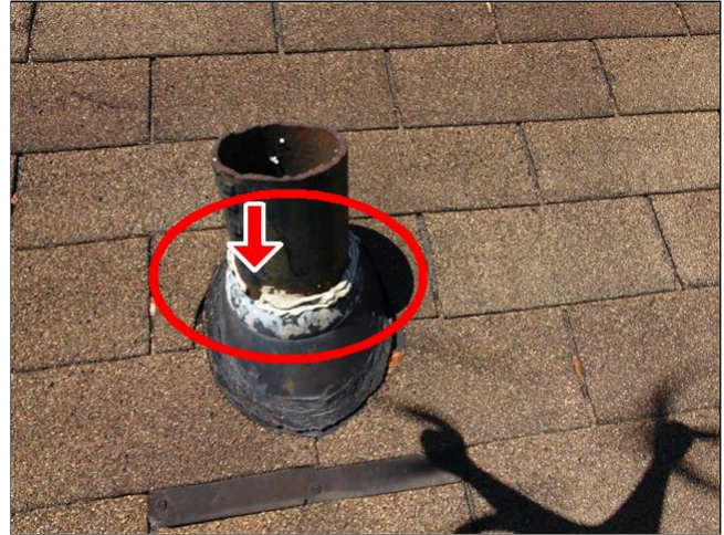
8.2 Item 2(Picture) Temporary Sealant and Openings
