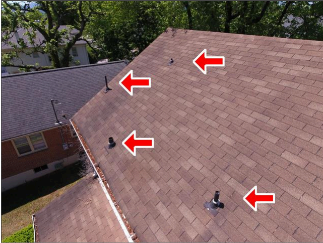
8.2 Item 1(Picture) Vent Pipes
