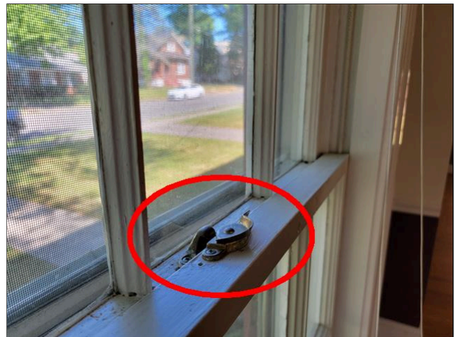
1.6 Item 4(Picture) Locks Don't Align (Multiple Windows)
