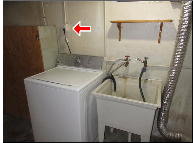
4.5 Item 2(Picture) Basement Laundry Area
