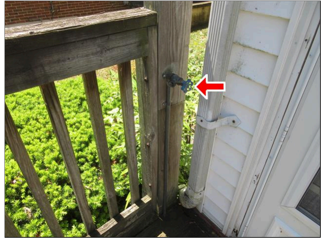
3.2 Item 4(Picture) Rear Deck
