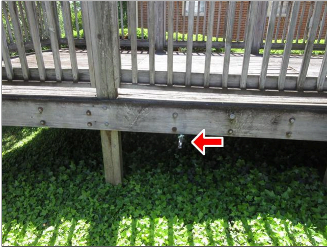
3.2 Item 3(Picture) Rear Deck
