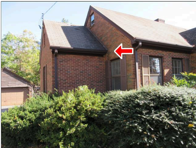
8.1 Item 1(Picture) Front Left
