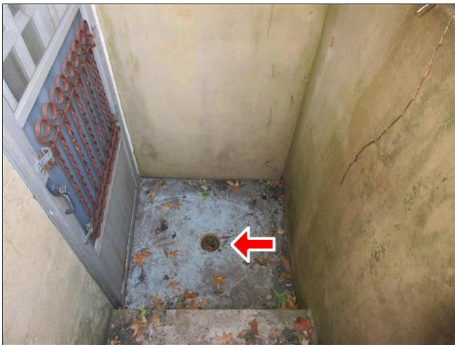
9.4 Item 1(Picture) Stairwell Drain
