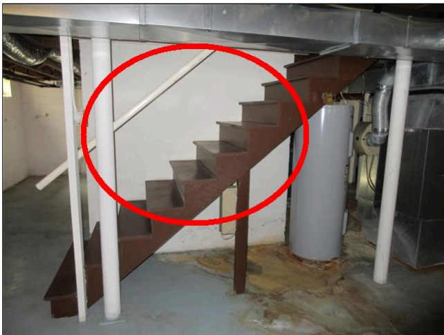
1.3 Item 1(Picture) Basement Stairs
