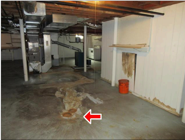
9.4 Item 3(Picture) Basement Floor Drain
