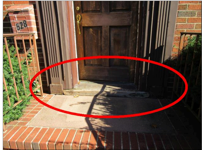
9.0 Item 6(Picture) Around Front Entrance
