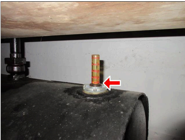
3.4 Item 1(Picture) Empty Oil Tanks
