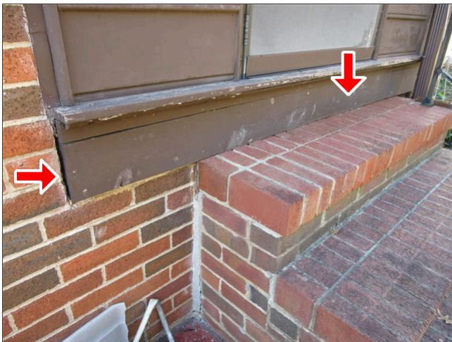
9.0 Item 3(Picture) Openings (Around Rear Door)
