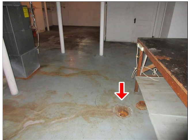
9.4 Item 2(Picture) Basement Floor Drain
