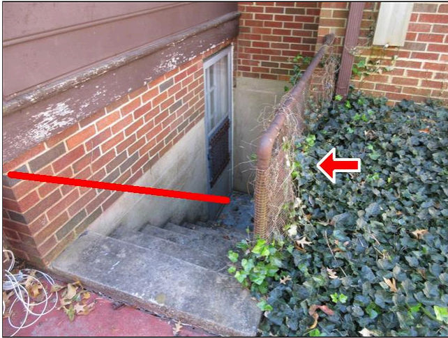
9.3 Item 1(Picture) Basement Stairs
