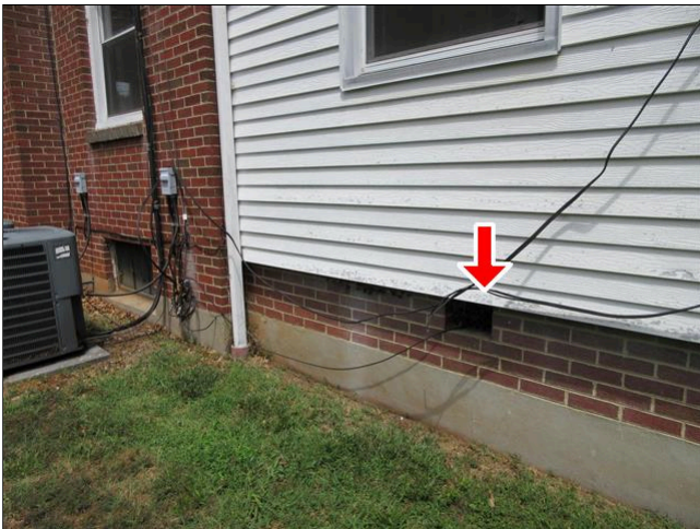
7.3 Item 1(Picture) Crawl Space Vents (Both Sides)
