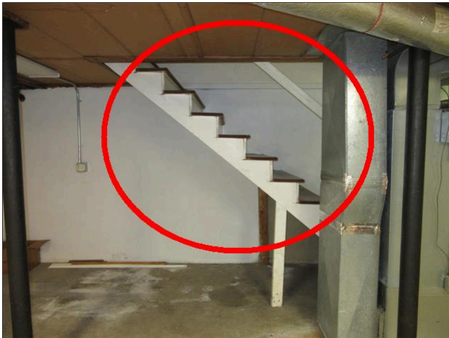
1.3 Item 1(Picture) Basement Stairwell
