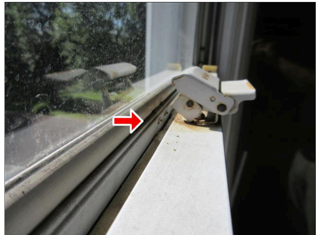
1.6 Item 4(Picture) Additional View
