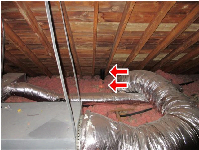
8.2 Item 3(Picture) Daylight (Attic View)
