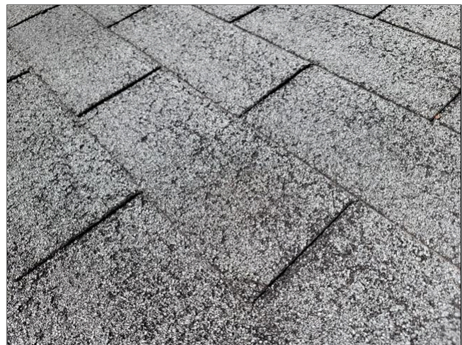
8.0 Item 4(Picture) Blistering, Brittle and Thinning Edges
