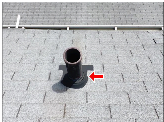
8.2 Item 2(Picture) Additional View
