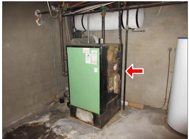
2.0.B Item 2(Picture) Old Abandoned Boiler
