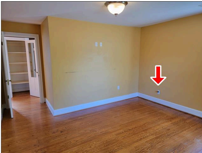
4.4 Item 1(Picture) Reversed Polarity (Upstairs Front Right Bedroom)
