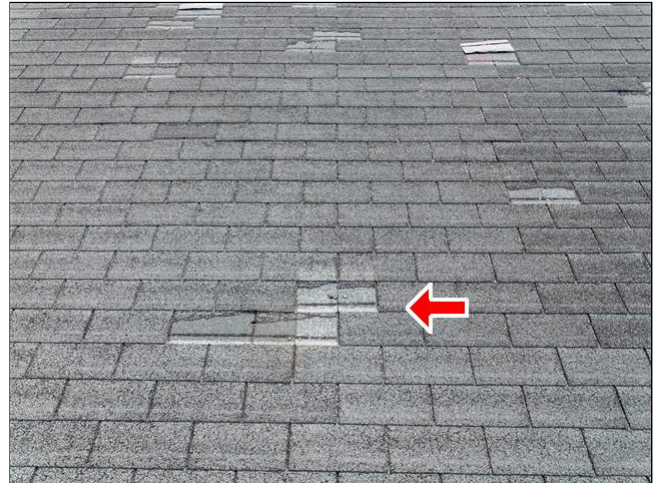
8.0 Item 2(Picture) Additional View
