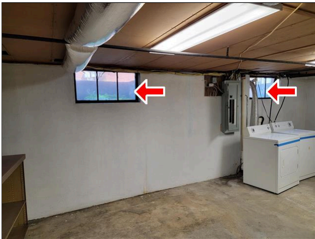
1.6 Item 1(Picture) Basement (Left Wall)
