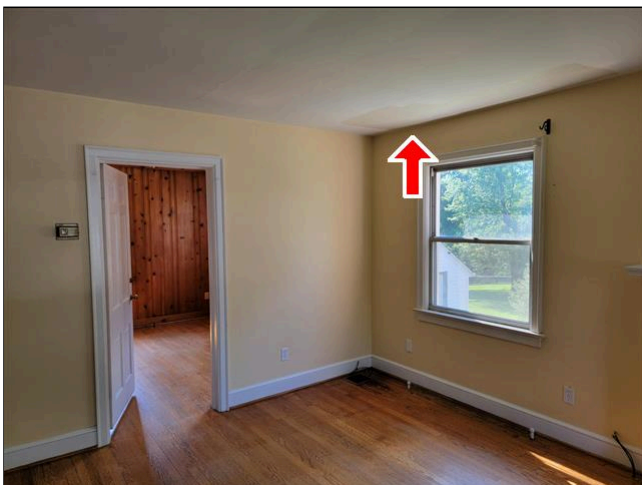
1.0 Item 3(Picture) Living Room (Under the Bathroom)
