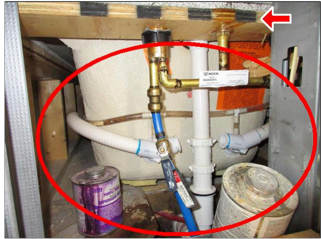
1.1 Item 2(Picture) Behind Wall Cavity
