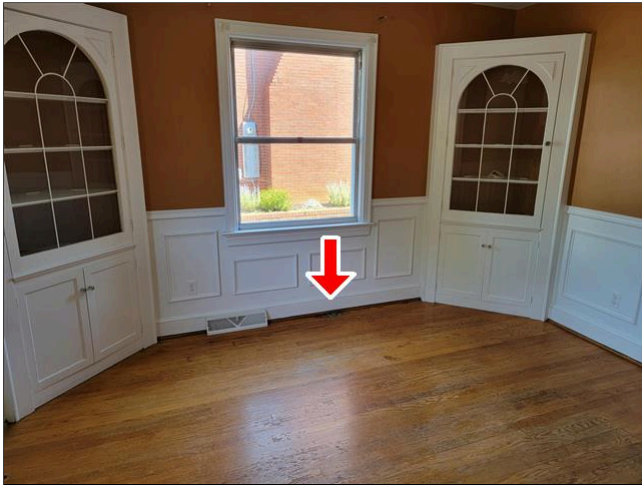
4.4 Item 5(Picture) Inactive Outlet (Dining Room)
