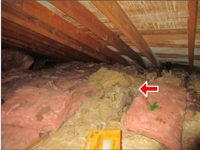
7.4 Item 1(Picture) Kitchen Exhaust Discharge (Under the Insulation)
