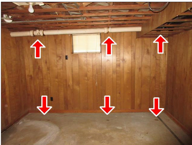
3.0 Item 1(Picture) Staining and Drips (Multiple Locations)
