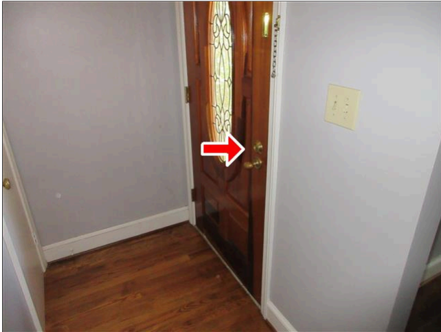
9.1 Item 5(Picture) Double Cylinder Lock (Front)
