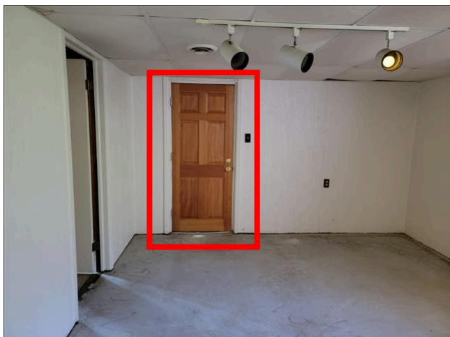
9.1 Item 3(Picture) Openings (Basement Entrance)
