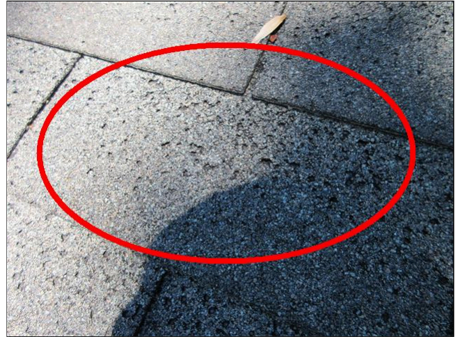
8.0 Item 2(Picture) Shingle Blistering (Multiple Locations)
