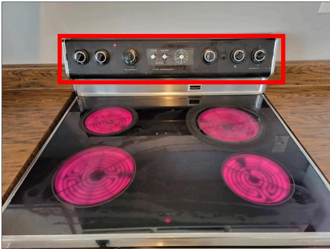
5.1 Item 1(Picture) No Control Panel Lettering Indicators
