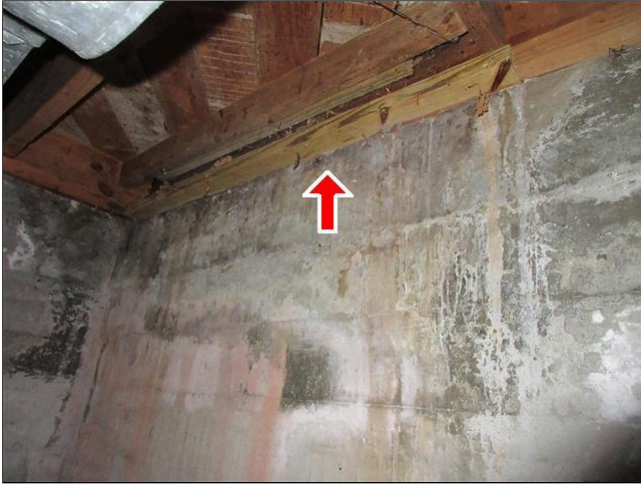
1.9 Item 3(Picture) Sill Plate Repairs
