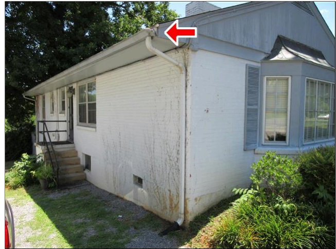
8.3 Item 4(Picture) Bent (Front Left)
