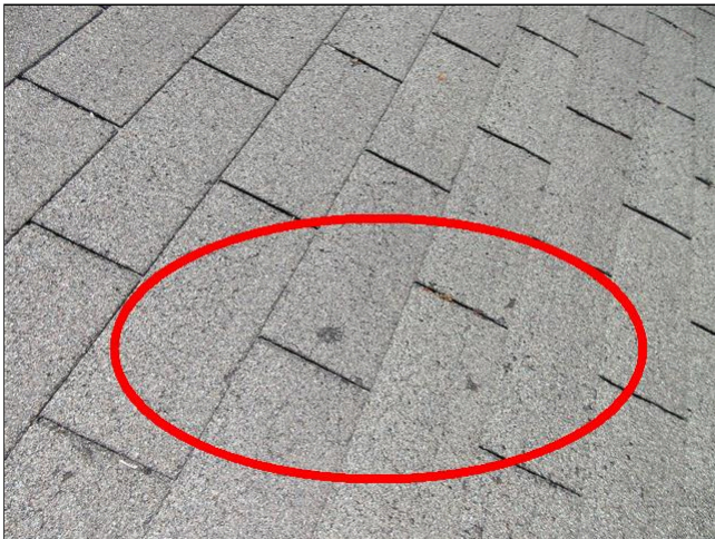
8.0 Item 3(Picture) Potential Hail Impact (Multiple Locations)
