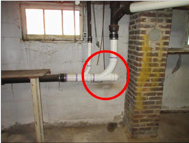
3.0 Item 5(Picture) Support Strap and Sagging Line
