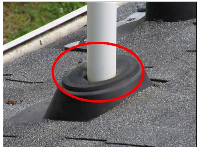
8.2 Item 2(Picture) Rolled Seal
