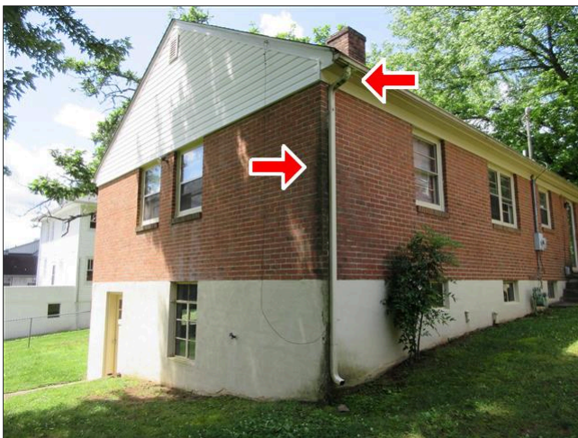
8.3 Item 3(Picture) Overflow Indications and Overgrowth
