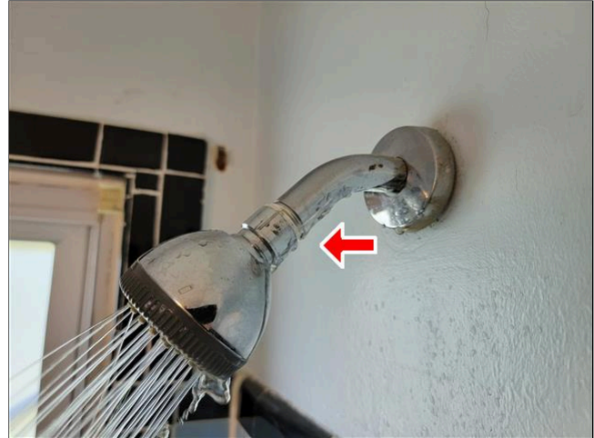
3.2 Item 11(Picture) Additional View
