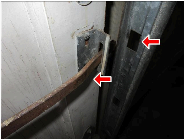
10.2 Item 1(Picture) Bent Lock Guides (Both Sides)
