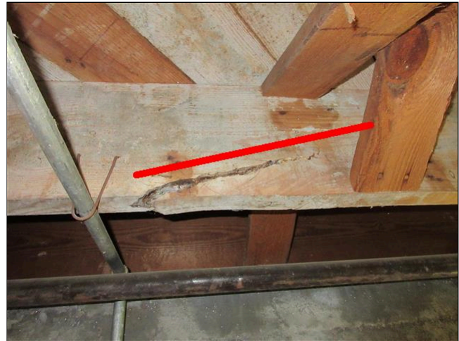
6.2 Item 2(Picture) Additional View
