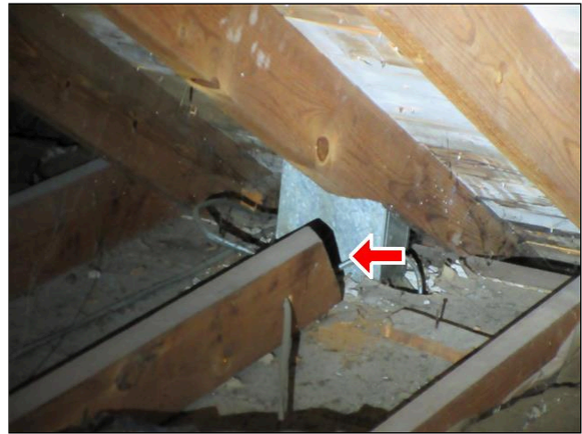
6.4 Item 2(Picture) Additional View
