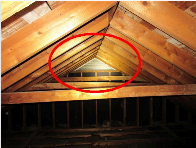
7.2 Item 1(Picture) No Screen (Front and Rear)
