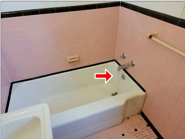
3.2 Item 4(Picture) Primary Bathroom
