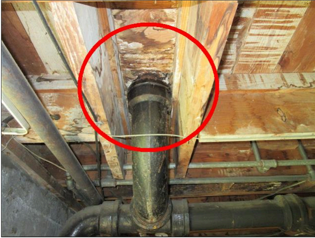
3.2 Item 3(Picture) Additional View
